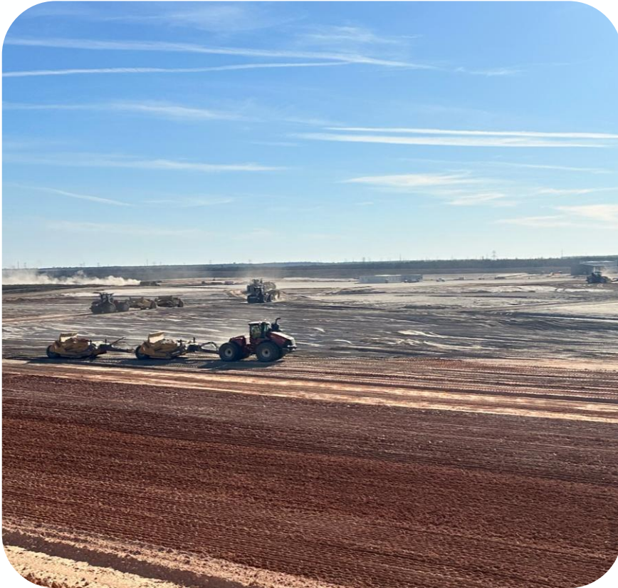
G2_AUSTIN CONSTRUCTION IN JAN. 2026
